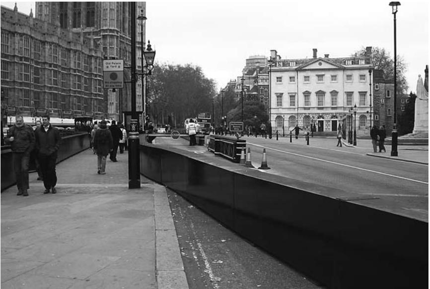
**Figure 10.8** Reinforced bi-steel barriers outside the Houses of Parliament
